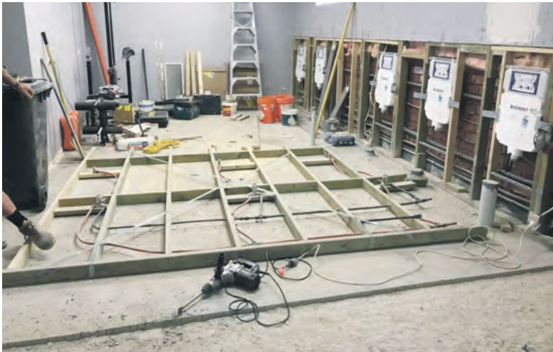
The change room upgrades are already under way and making great progress.
