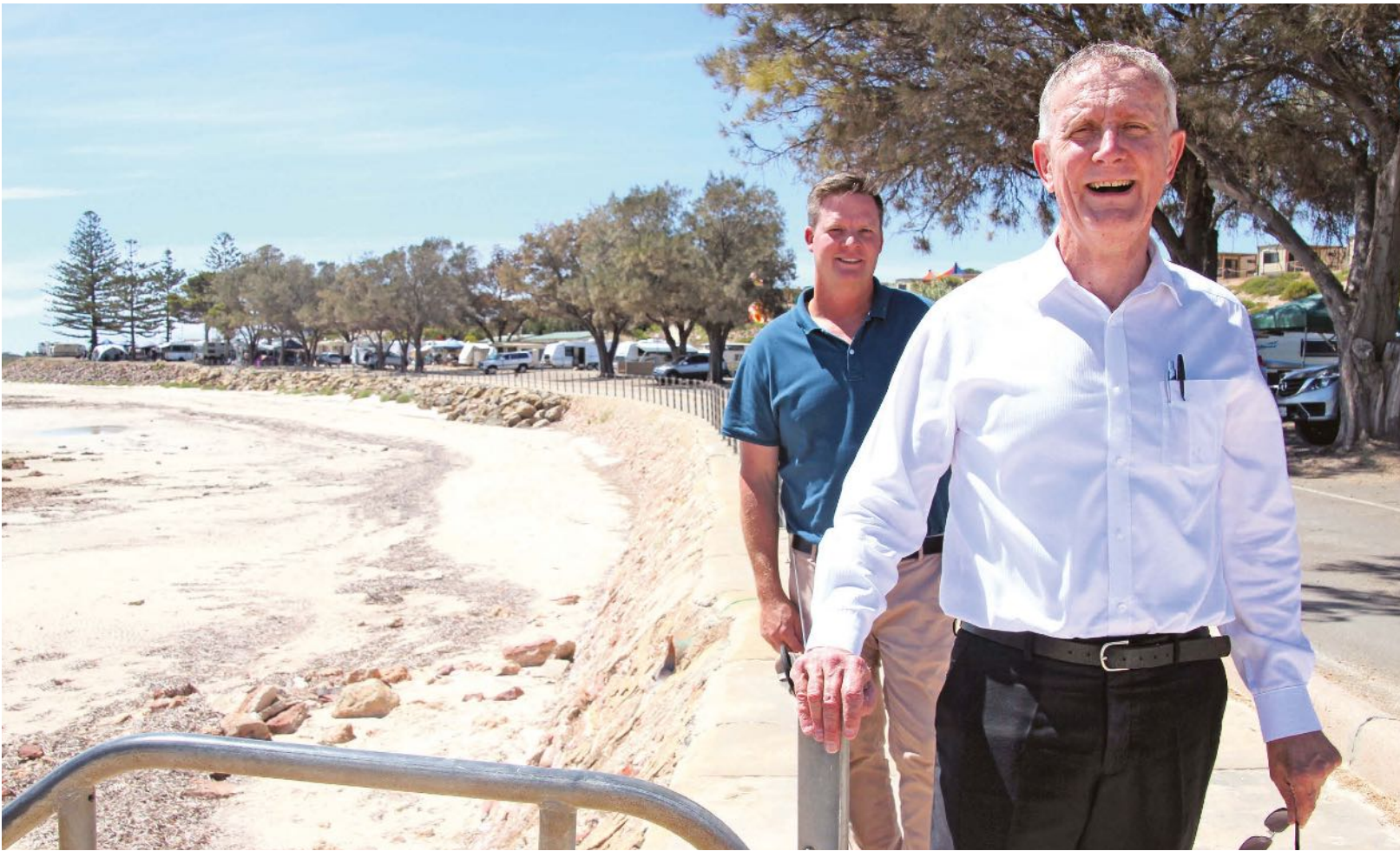
ROCK ARMOURING... Copper Coast Council CEO Russell Peate (front) and director of infrastructure services Tim Neumann are pleased to start work on the Moonta Bay foreshore rock armouring project, funded by a Regional Coastal Protection Grant.
